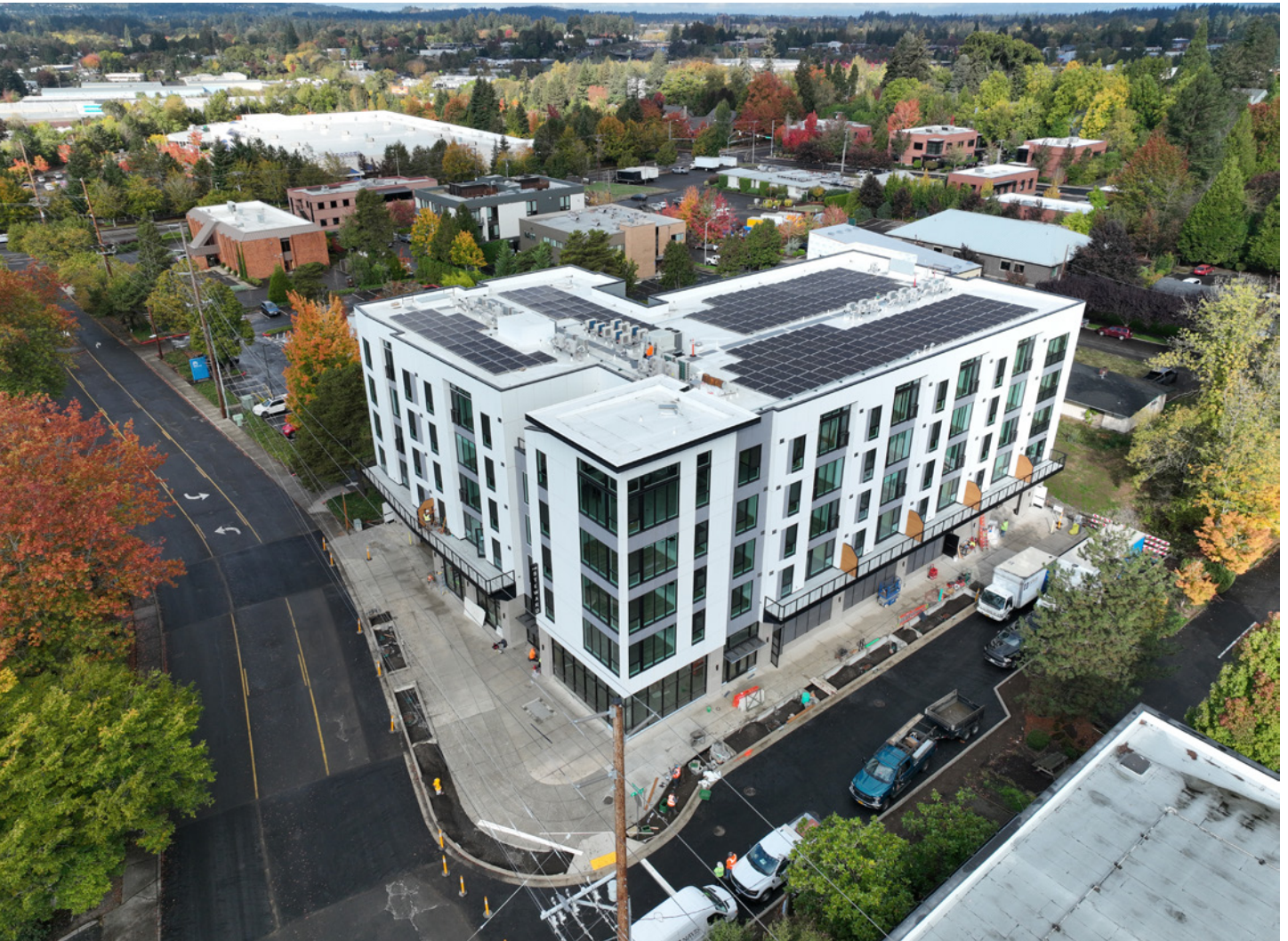
Crews are almost finished constructing The Steward – a five-story building in Tigard that has a rooftop solar array. (courtesy of DIG Real Estate)
