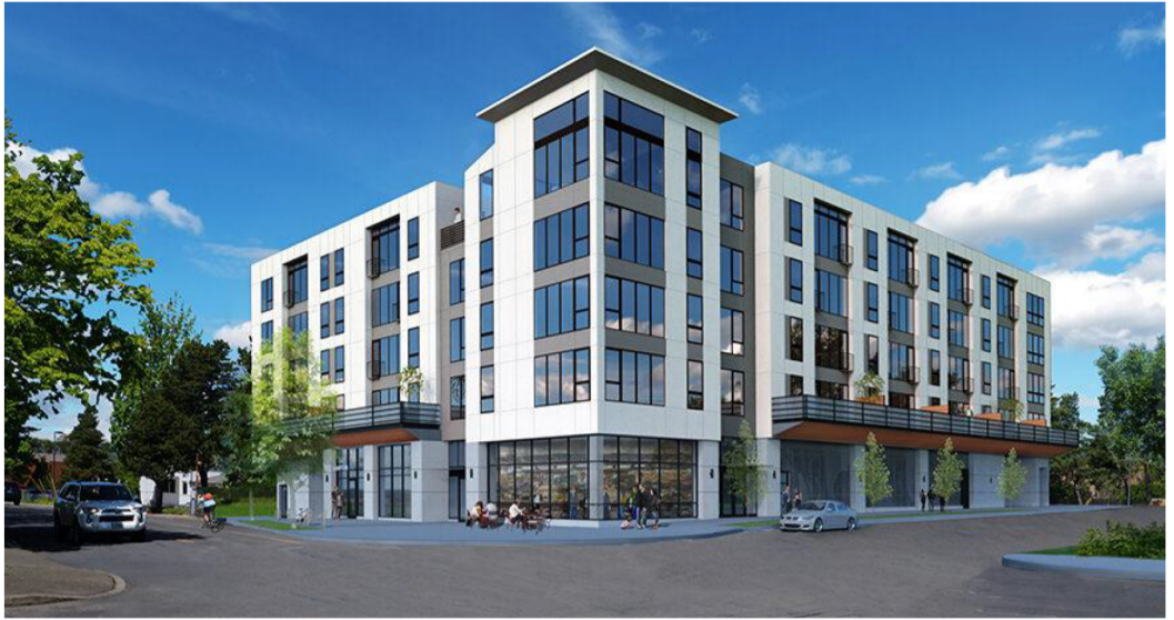
A five-story building under construction in Tigard will have 55 apartments. (courtesy of Leeb Architects)
