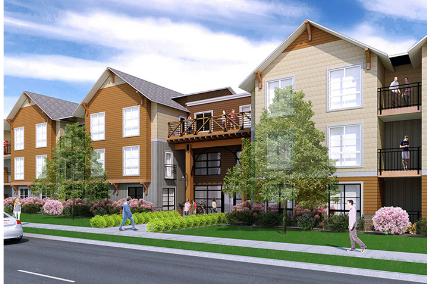
A new apartment complex in Fairview will contain 200 units on a 4.8-acre site. (Courtesy of Leeb Architects)
